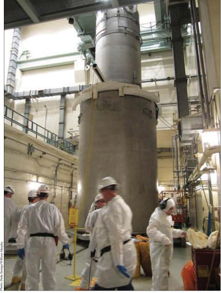
Workers at the Duke Energy-operated Catawba plant prepare the Transportable Storage Canister for transfer into the Vertical Concrete Cask. This ultra-high capacity dry cask storage system lowers employee radiological exposure, stores more used fuel, reduces the number of containers needed, and saves the company millions of dollars.
