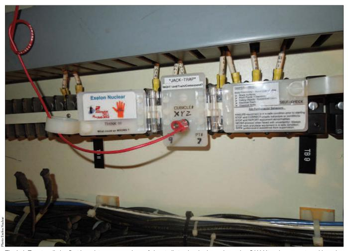
The Jack Trap, installed at Braidwood, is constructed out of electrically insulated nylon and tested to 5 kV. Hinged construction adds to the portability and ease of installation.
