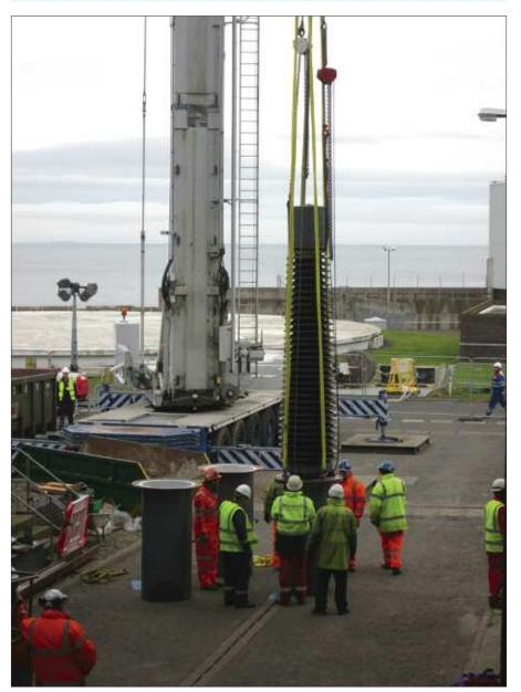
Torness-I's transformer bushings are lowered to the ground outside the Unit I reactor building.
