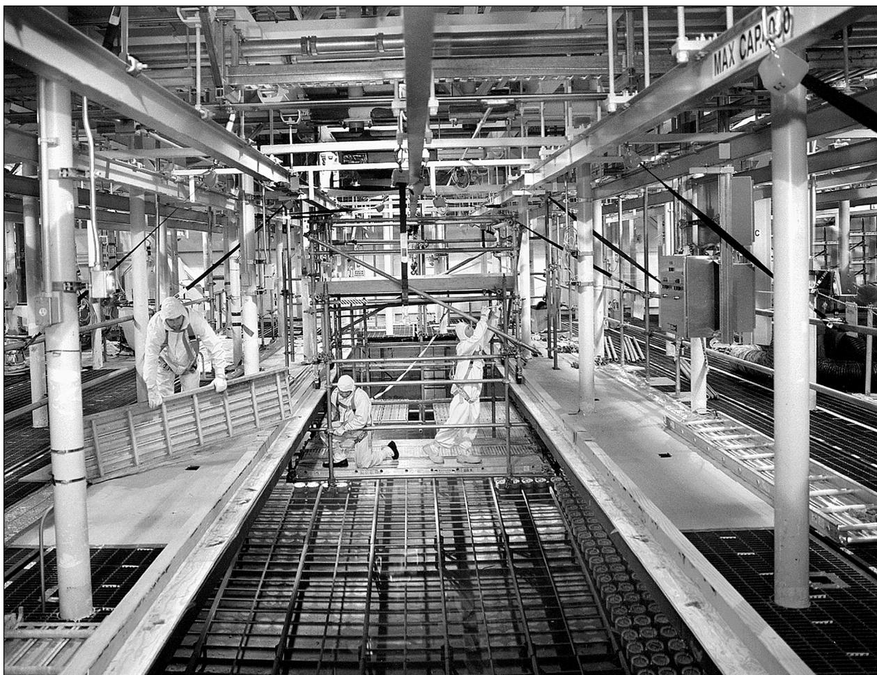
Removing K-West floor grating to make room for fuel-removal equipment.
