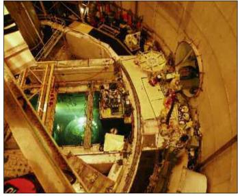
**Left:** Siempelkamp's tooling cuts the lower core barrel during the final stages of Unit 2 reactor vessel internals segmentation. **Right:** A view from above of the deep end of the Unit 2 reactor cavity shows the lower internals undergoing segmentation.
