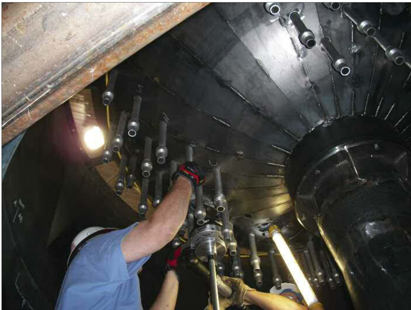
Workers use the mock-up to practice machining activities at Calvert Cliffs. (Photos: CENG)
