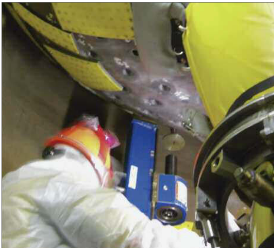
A worker machines the pressurizer to accept the new heater sleeve.
