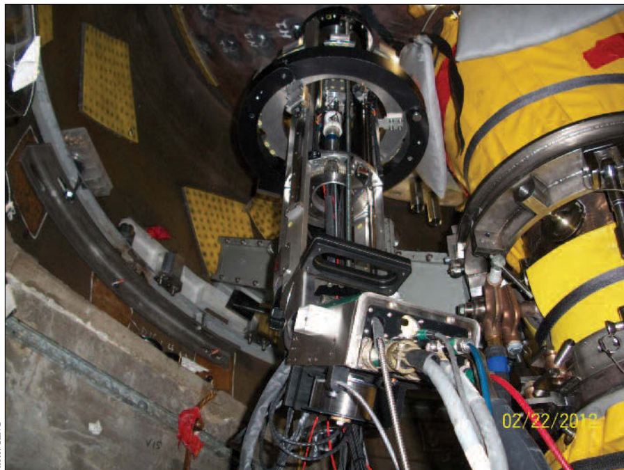
Best of the Best: At Calvert Cliffs, the remote weld head delivers the new stainless steel heater sleeve. Once the sleeve is delivered, the weld head is used to make the ID Temper Bead weld of the sleeve to the pressurizer.
