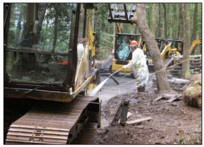
Power washers ensured the removal of any radioactive contamination clinging to heavy equipment used to remove soil near Lower Three Runs at SRS. The equipment was then radiologically surveyed to confirm acceptable release limits were met.
