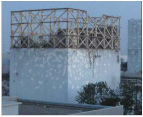
Unit I at the Fukushima Daiichi nuclear power station on March 12, 2011, following the earthquake and tsunami and after an explosion that opened up the top of the outer reactor building's shell . . .
