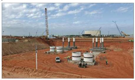
This shot of the Vogtle new construction site, taken on November 3, 2011, shows circulating water system pipes that will connect to Unit 3's turbine building and condenser. (Photo: Southern Company)
