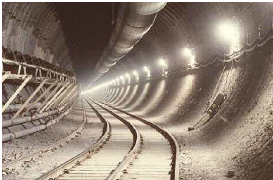
The interior of Yucca Mountain's main tunnel (Photo: DOE)
