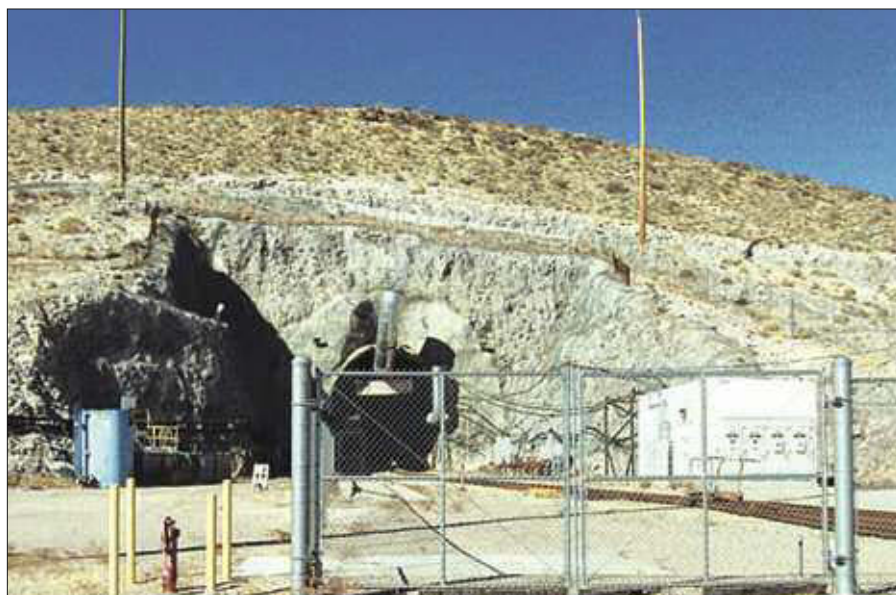
The Yucca Mountain north portal tunnel entrance (Photo: GAO)
