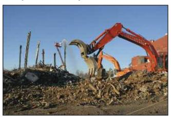
Building 9211 D&D almost complete, with excavator removing rubble from building site.
