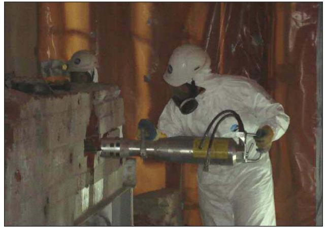
Coring and bursting operations of an "instrument bulge" (historically used to extract process liquor for analysis in the Primary Separation Plant) prior to removal from the facility.
