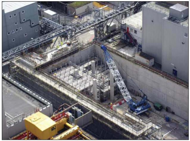
Progress as of mid-April 2010 on the Sludge Packaging Plant at Sellafield, which will receive legacy sludge from the First-Generation Magnox Fuel Storage Pond.
