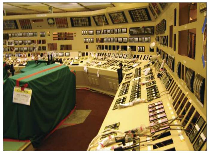
The Watts Bar-2 control room will maintain continuity with the controls and procedures in effect for Unit 1. It may have been possible to convert Unit 2 entirely to digital instrumentation and controls, but TVA prefers that Unit 2 be operable in the same way as Unit 1.
