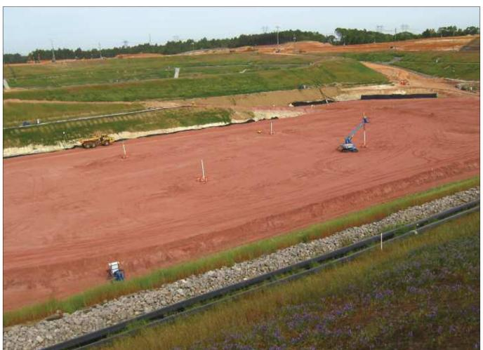
The Vogtle-3 excavation contained about 8 feet of backfill at the time of this photo (April 19). The slopes surrounding the excavation are terraced every 30 feet of height, with ramps to allow equipment to enter and leave.
