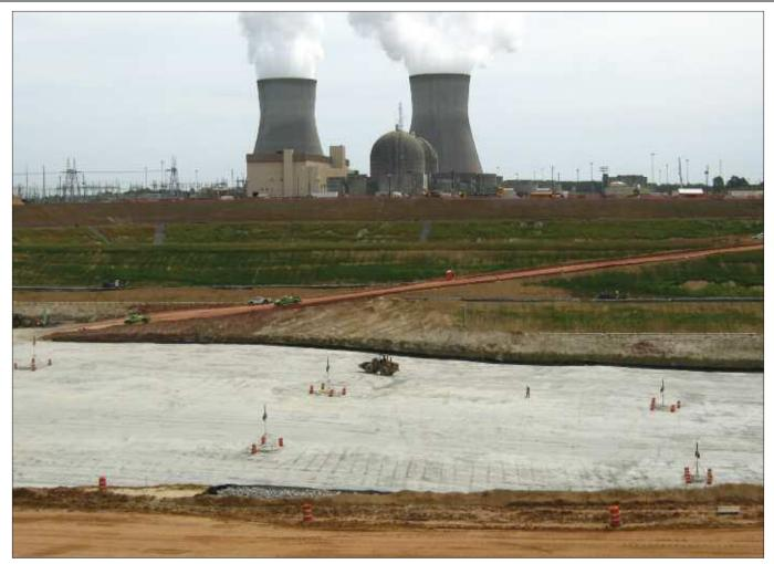
On April 19, backfilling had not yet begun for Vogtle-4. The structures on the blue bluff marl measure the vertical motion of the rock; with the 90-foot depth of dirt removed, the marl had risen measurably, and it was expected to lower again once the backfill was placed. Units I and 2, both in operation at the time, are in the background.
