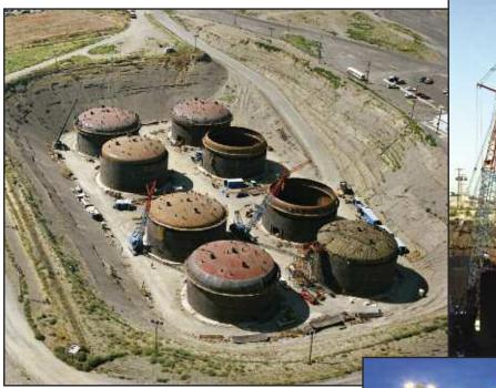
Underground tanks were constructed to hold radioactive and chemical wastes from nuclear weapons activities. At the Hanford Site, 177 underground tanks were built, and more than 60 of these have leaked or are suspected of leaking waste to the surrounding soil.
