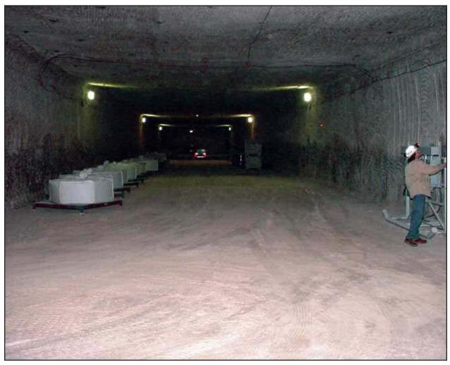
A newly ready disposal room in Panel 3 showing width and height before significant closure begins. Note the comparative lack of roof bolts.
