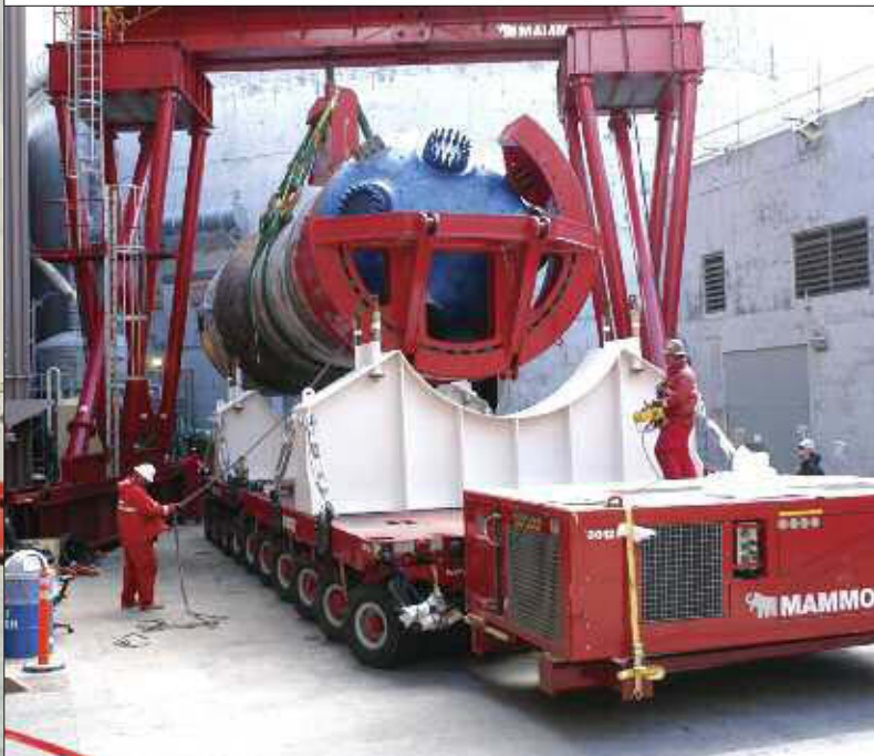
A failure-proof, seismically qualified single-point lift system (left photo) was used to pick up each steam generator and place it on a heavy transporter (right photo).
