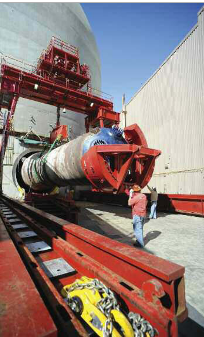
A failure-proof, seismically qualified single-point lift system (left photo) was used to pick up each steam generator and place it on a heavy transporter (right photo).
