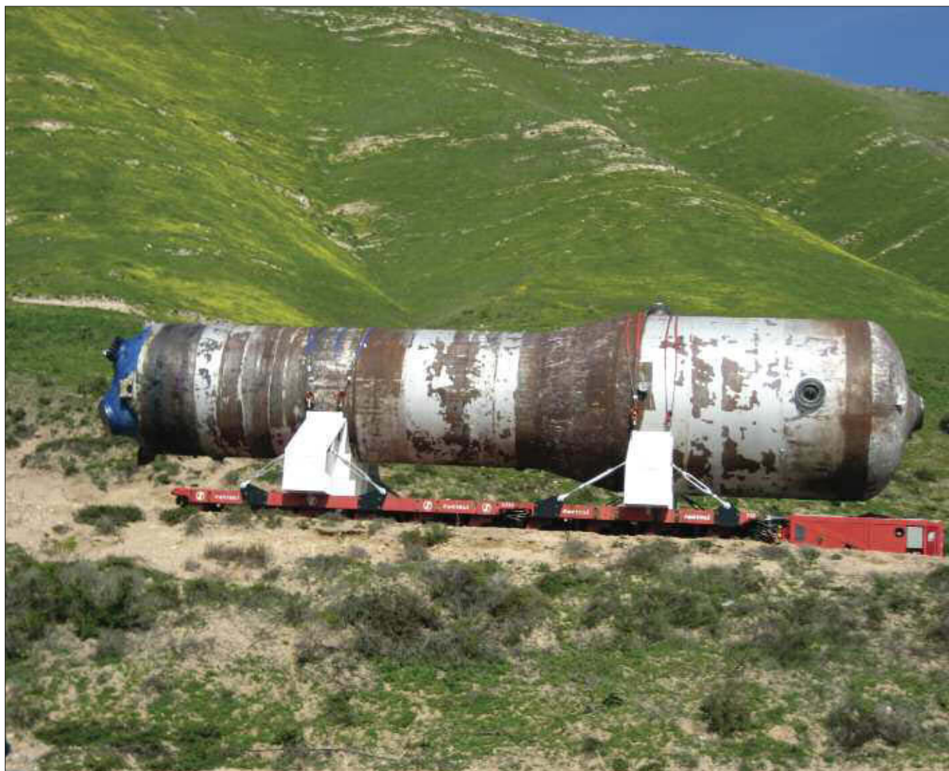
Each old steam generator was delivered by a truck transporter to a railcar, then carted by rail line uphill to the on-site storage building.
