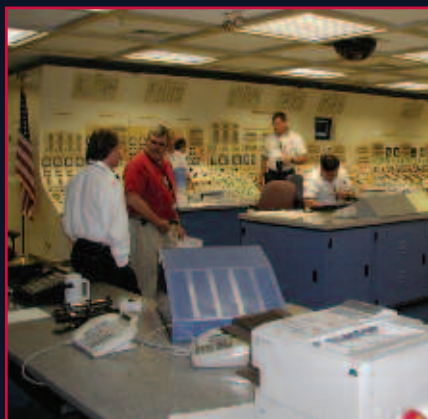
South Texas Project Simulator
