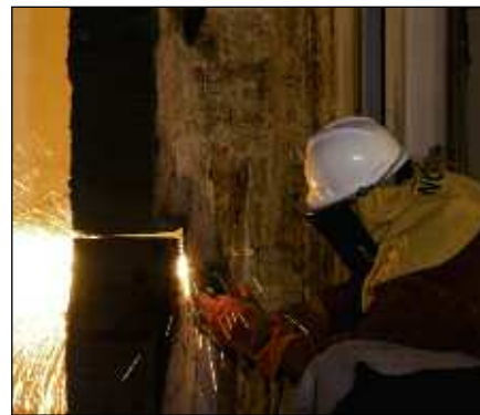
Cutting through P Reactor's steel doors at the Savannah River Site. The article beginning on page 40 looks at the P Reactor closure work.
