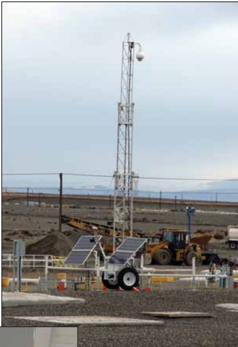
Above: Movable camera systems monitor single-shell tank farms where no work is being done. These systems can be moved to any location in the tank farm complex.
