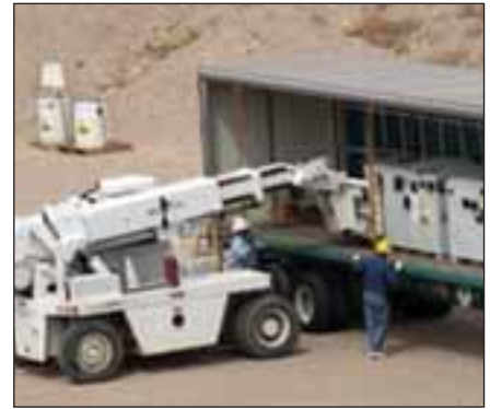
Disposal of mixed LLW packages at Pit 3 at the Nevada Test Site. See article beginning on page 56 for details.
