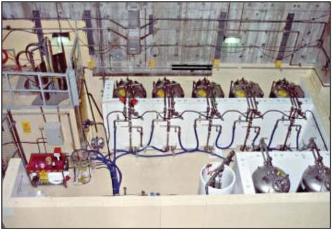
Fig. 2. Typical in-service filtration demineralizer system.
