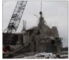
The concrete once hidden inside the distinctive Big Rock sphere was almost down to grade in mid-December at the Big Rock Point Restoration Project. A photo essay beginning on page 46 looks at a controlled demolition project at the
