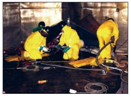
Working on diamond wire in support of cutting reactor vessel muzzles (launderable protective clothing).
