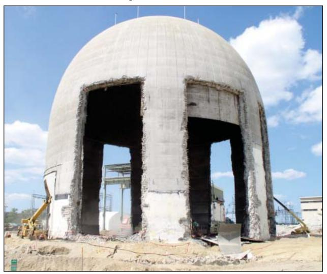
Hoe rams and cutting torches were used to cut the arches in the containment building.
