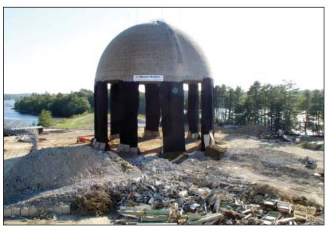
Eerily reminiscent of ancient temple ruins, the containment stands ready for the explosion, with the columns wrapped in fabric and chain-link fencing to minimize flying debris.
