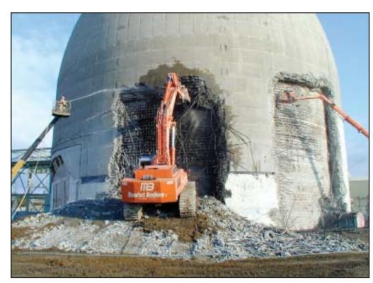
Pounding the concrete to create the arches.
