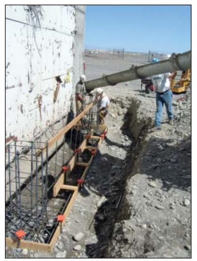
Chad Osbourne, left, and Rigo Rivas, right, pour a concrete footing for the structural steel to enclose a lead shield wall.
