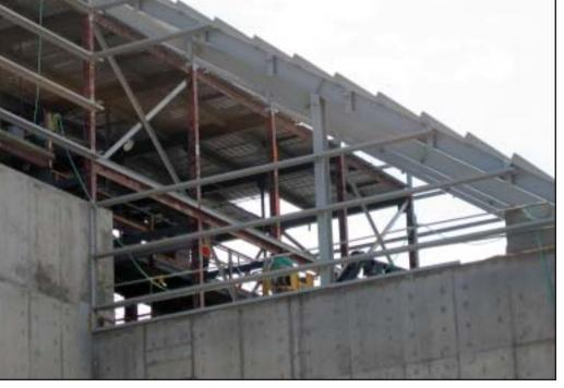
D Reactor roof frame shows how new steel was joined to old steel so workers can apply galvalum roof panels.
