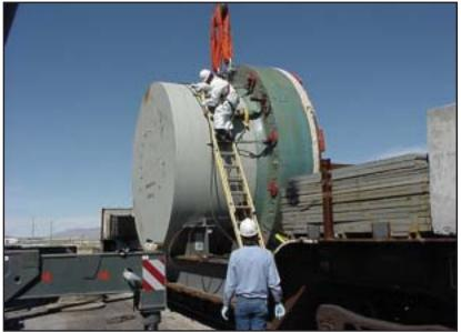
Davis-Besse reactor head being loaded onto depressed, flat railcar.
