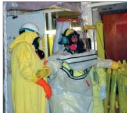
Suiting up at Rocky Flats. The article beginning on page 42 looks at the difficult D&D of the Site's Advanced Size Reduction Facility.
