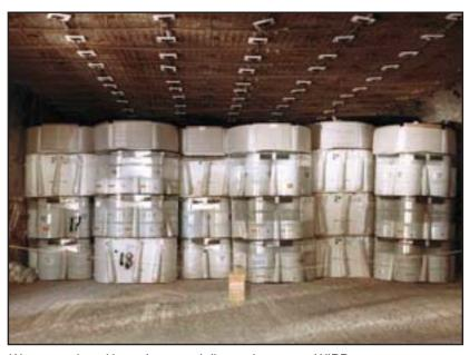
Waste emplaced in underground disposal rooms at WIPP.
