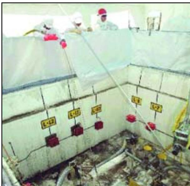
*Compared to baseline pit operations methods shown here, remote systems will reduce worker exposure and enable more thorough removal of discarded materials in Hanford pump pits. (Photo courtesy ORP.)*
