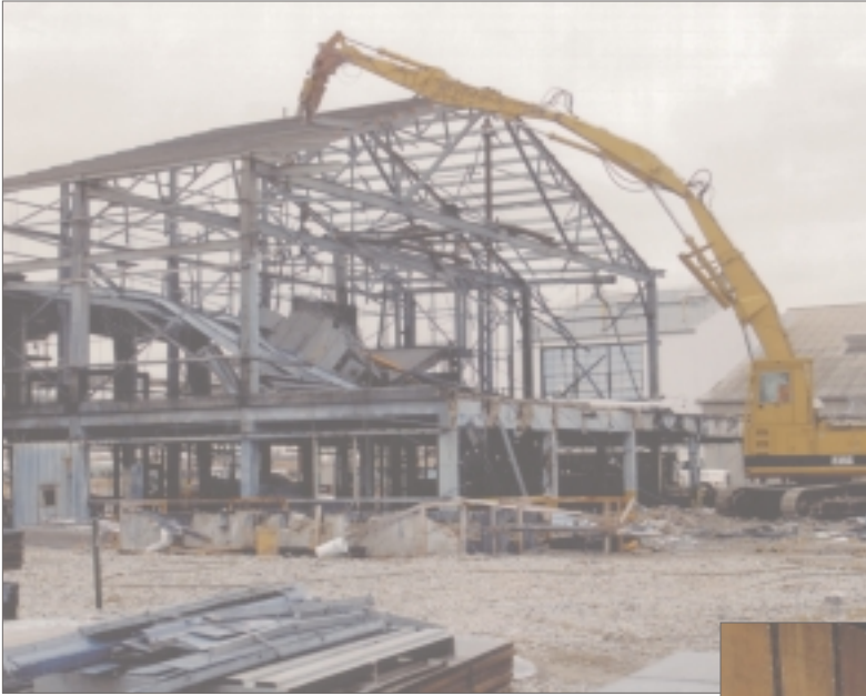
Dismantling a building at Fernald.
