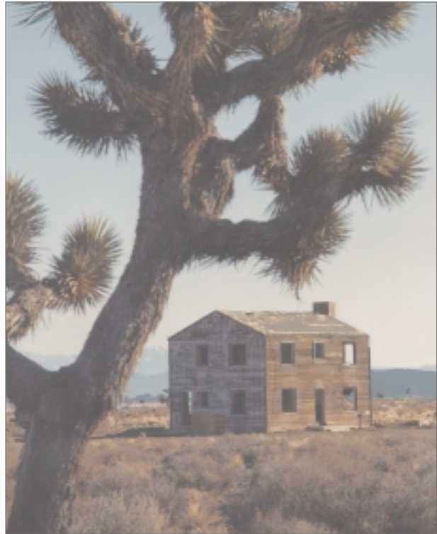
This "Survival Town" house remains standing on the site. Survival Town was built for a Civil Defense exercise and to test items not previously subjected to a nuclear blast. It consisted of houses, office buildings, fallout shelters, power systems, communication equipment, a radio broadcasting station, and trailer homes. A 29-kiloton nuclear detonation a little over a mile from the town site was conducted in 1955.
