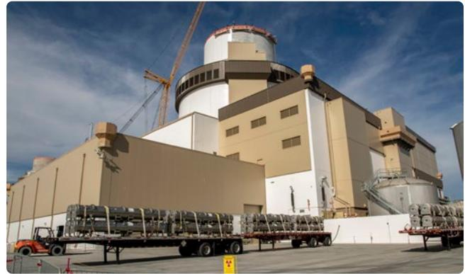
Fuel being prepared for unloading outside of Vogtle-3 in January. (Photo: Georgia Power)
