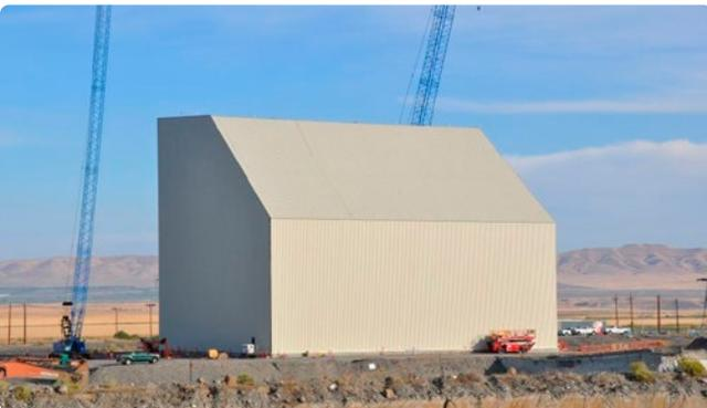
A protective steel cocoon was built over the former K East Reactor building at the DOE's Hanford Site. (Photo: DOE)
