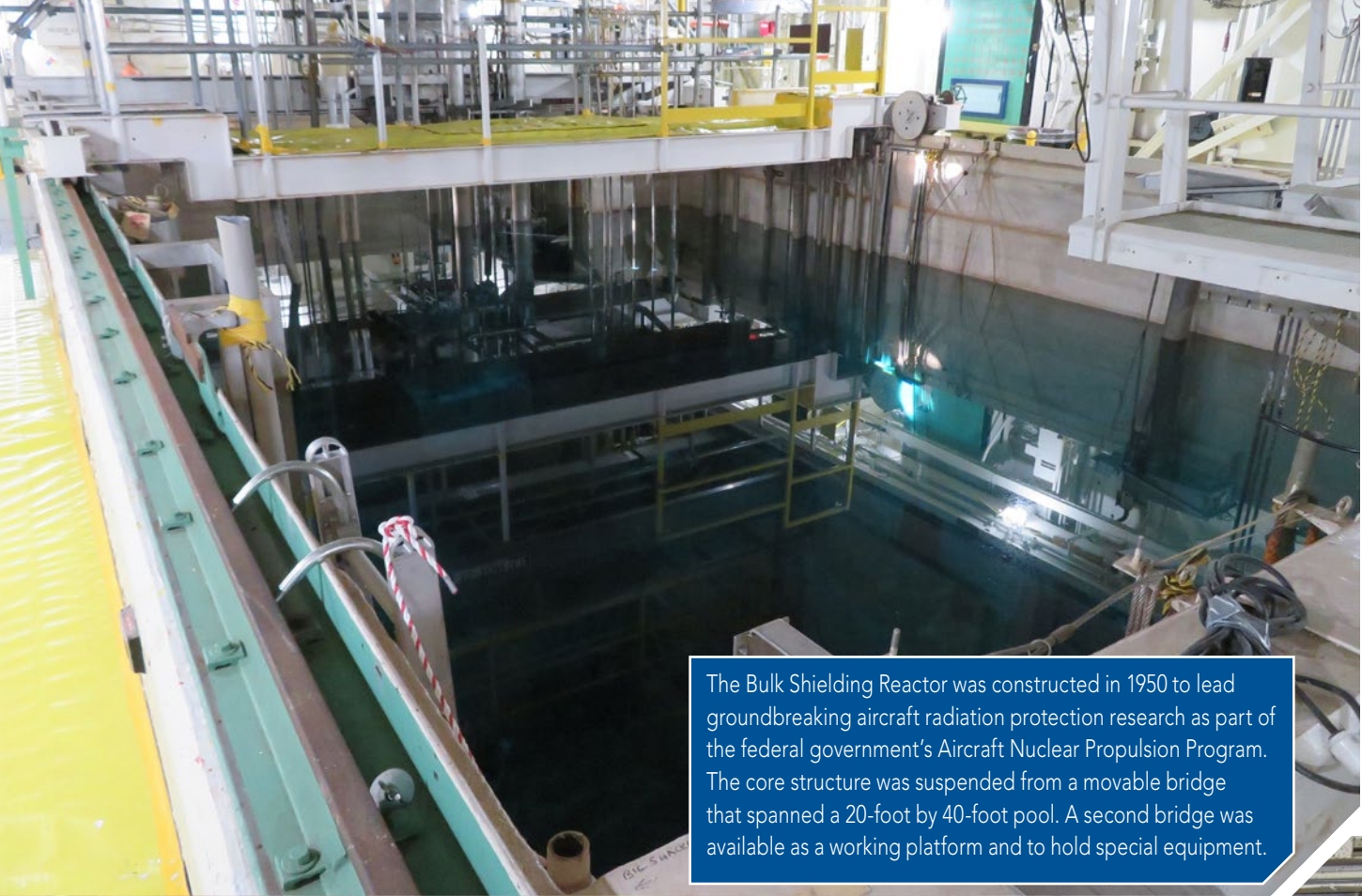
To prepare the 3010 Bulk Shielding Reactor building for demolition, the 27-foot-deep reactor pool inside the building was filled with a concrete mixture.
