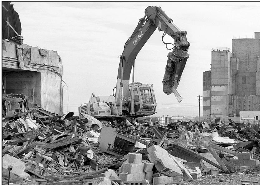
*Demolition began in February at Hanford's fourth plutonium production reactor to undergo the cocooning process and should be completed in fiscal year 2003. In the background is DR Reactor, where cocooning is 85 percent complete. The final step in the DR Reactor cocooning process is to install a new roof over the entire structure, which should be completed in fiscal year 2002. Hanford is home to nine surplus plutonium production reactors.*
