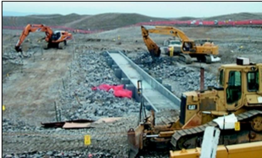
*Remediation of Hanford's 116-N-3 crib has been a major challenge. The restoration team spent nearly two years in planning the work to limit worker radiation exposure to as low as reasonably achievable. Before protective measures were implemented, radiation levels at the soil surface were as high as 500 mrem/h.*
