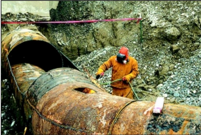
More than 17 000 ft of reactor effluent piping was removed from D and DR Reactors. Major challenges in excavating the 60-in.-diameter piping included containing contamination-bearing rust from inside the pipe and asbestos cladding from the outside.
