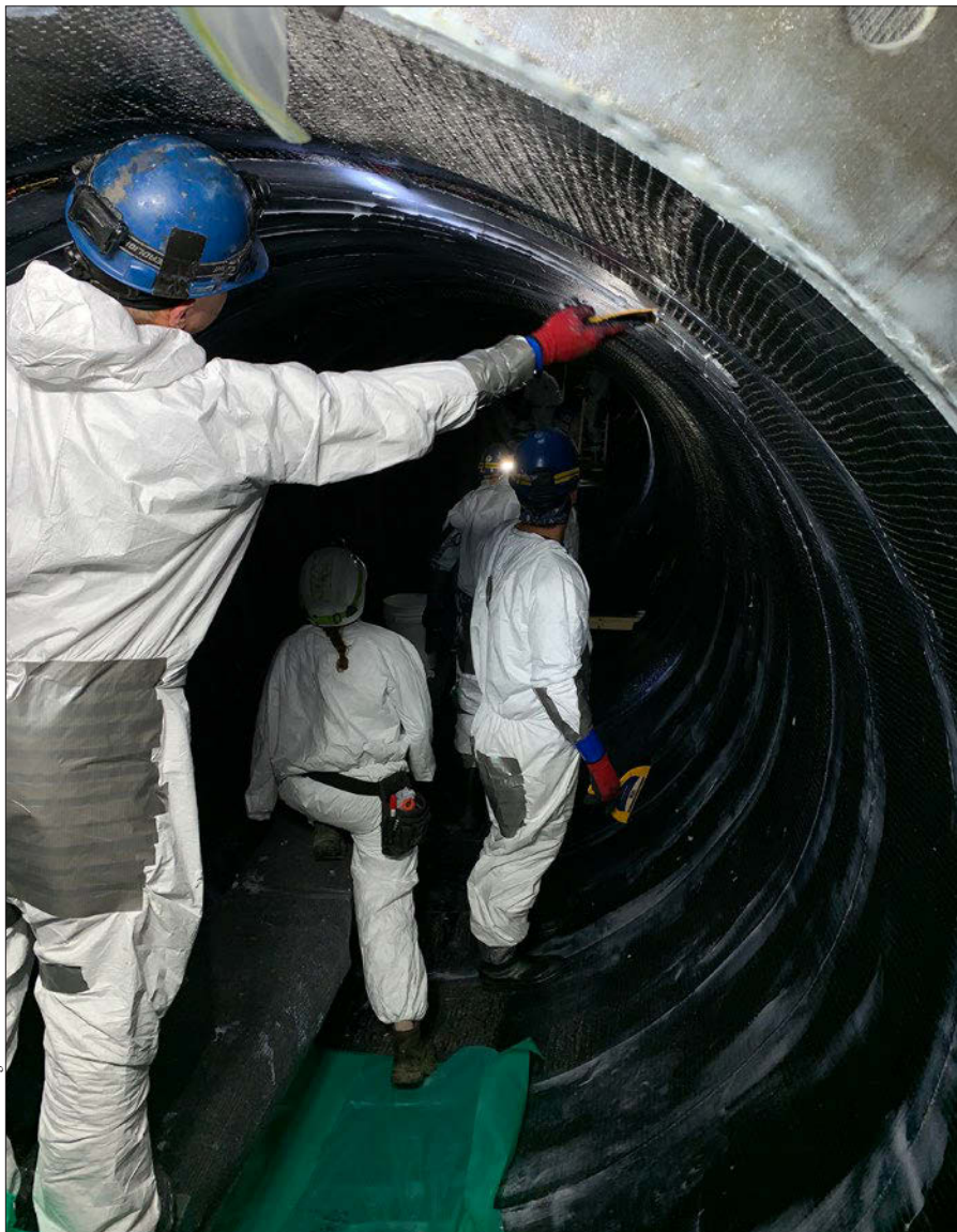
Quality control inspections were ongoing during the CFRP installation process as part of the pipeline upgrade.
