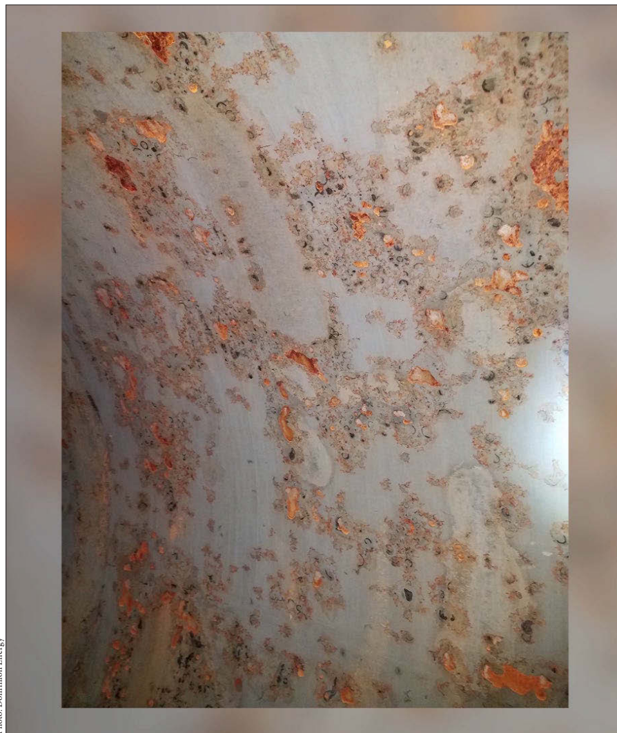
The condition of Surry’s metallic pipelines required routine repair work, driving the desire for a long-term CFRP upgrade.
