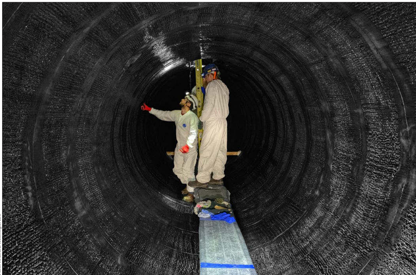
Quality control inspectors carry out a detailed post-installation examination of the installed CFRP lining system.
