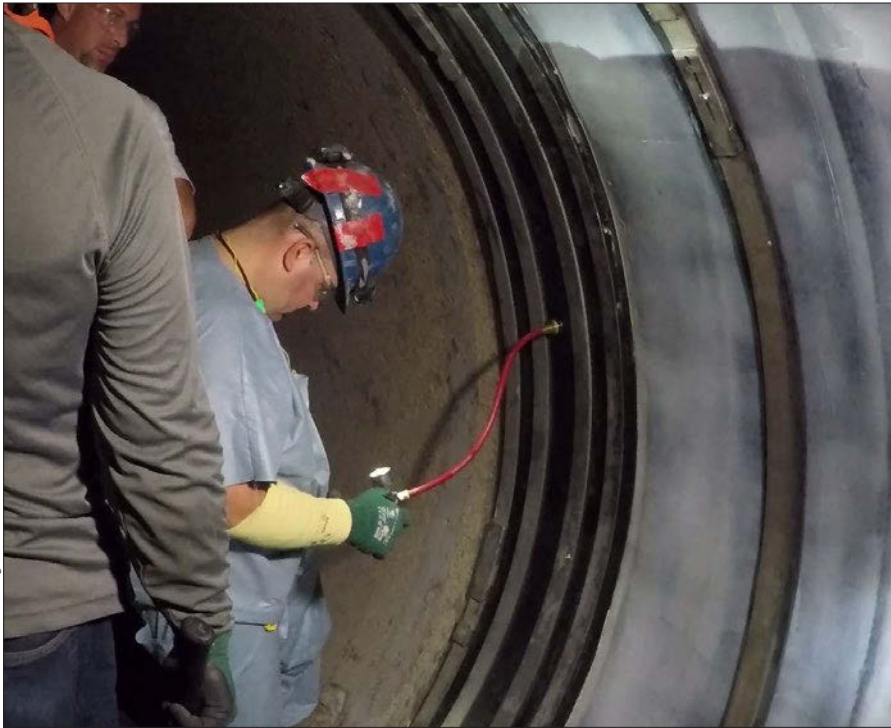
Custom-designed termination points are critical to the long-term performance of the CFRP lining system.
