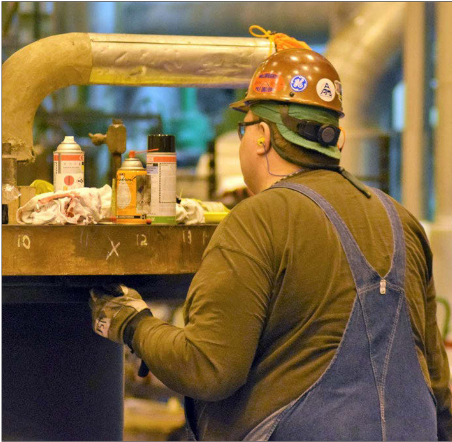
A General Electric technician cleans parts as his group begins to reassemble the Davis-Besse turbine.
