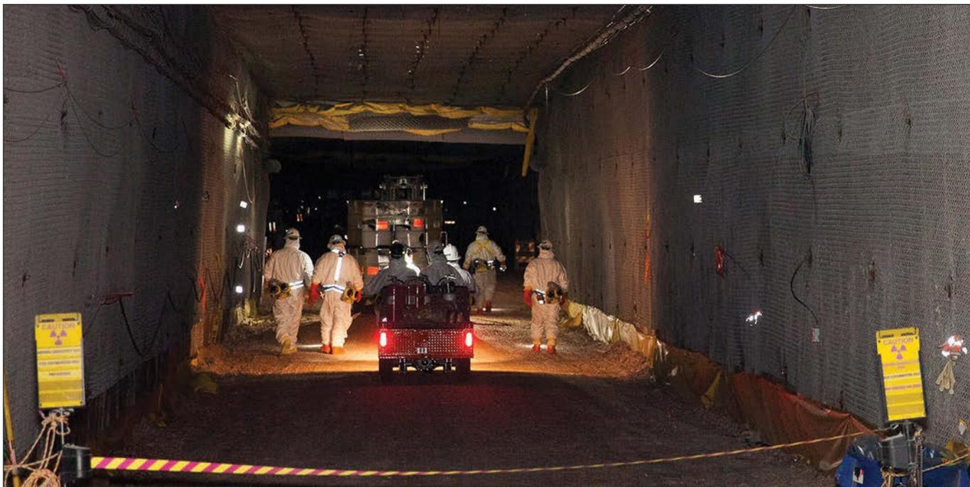
Workers at WIPP resume disposal operations, emplacing drums of waste in the underground on January 4. (Photo: DOE)
