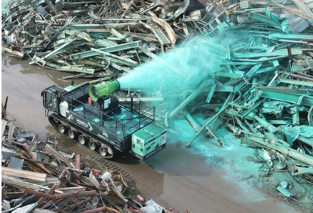
Above: The tracked Prinoth Panther T16 crawler carrier features a zero-degree turn radius and is able to adapt to irregular terrain. It traverses the X-326 demolition area daily, spraying fixative on building debris with an onboard Dust Demolisher and 2,700-gallon tank of fixative to lock down dust.
