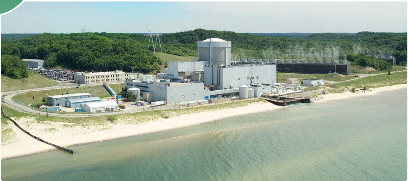
The Palisades nuclear power plant. (Photo: Holtec International)
