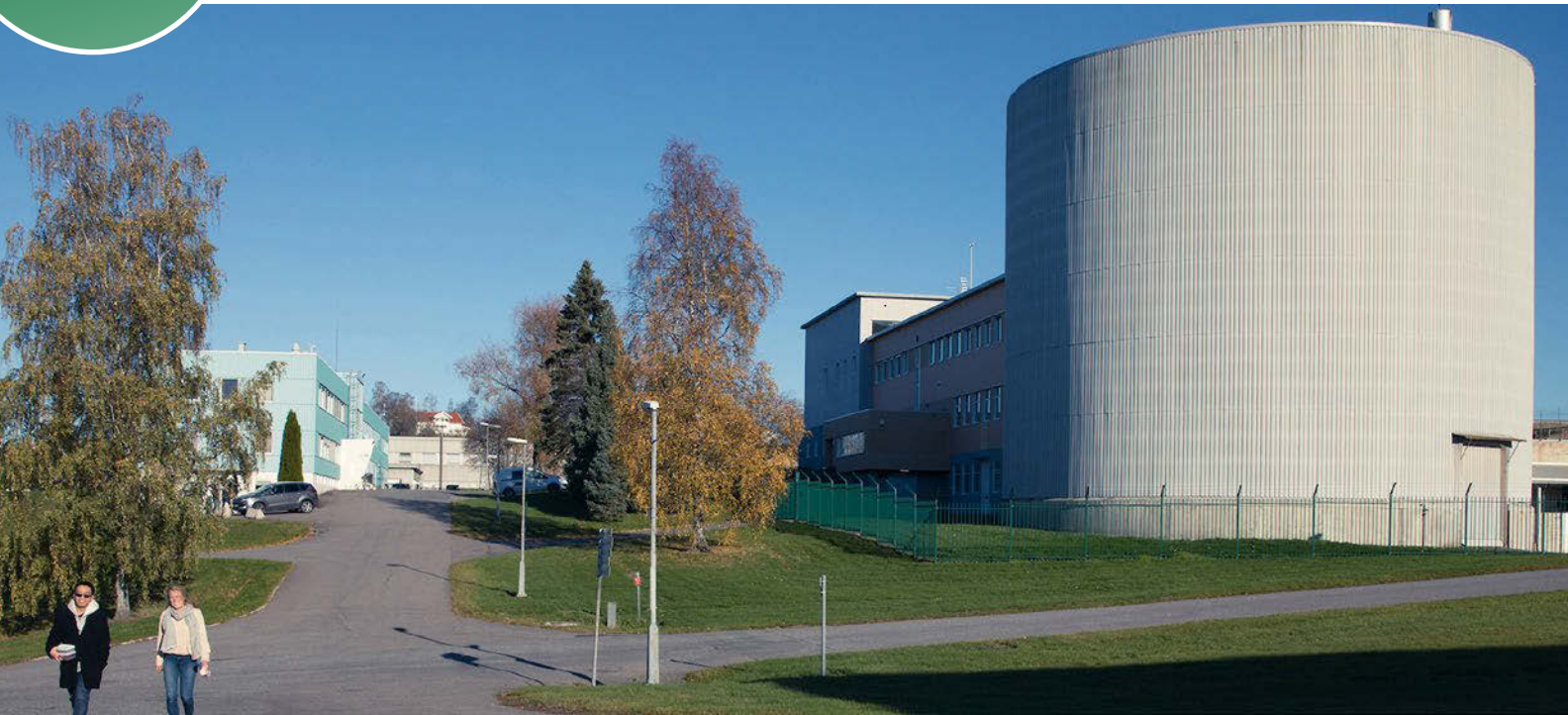
The JEEP-II facility at Kjeller, Norway. (Photo: Institute for Energy Technology)
