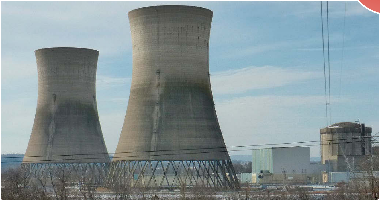
The cooling towers of Unit 2 at Three Mile Island Nuclear Generating Station, closed since the accident in 1979.
