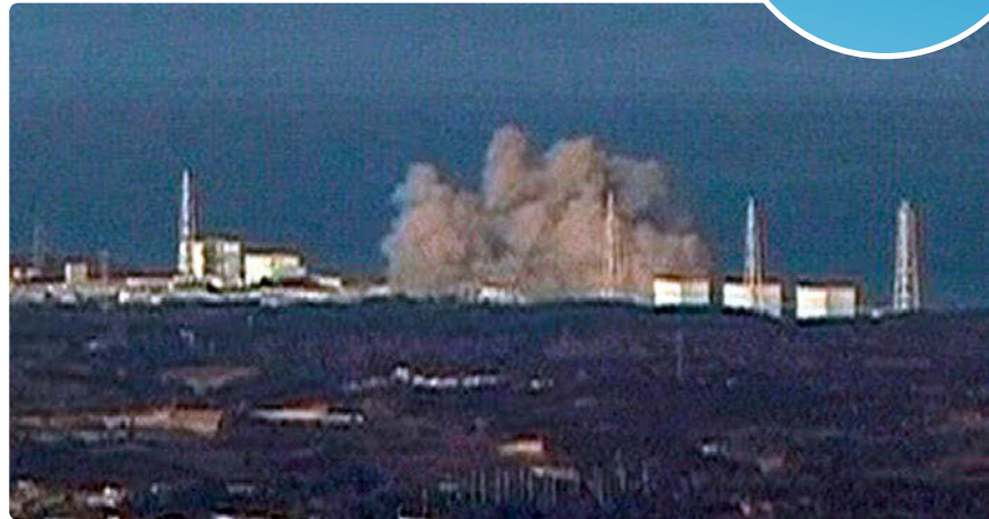
The explosions that spread material from the Fukushima meltdown were hydrogen gas explosions, not nuclear. (Photo: Wiki Fandom)
