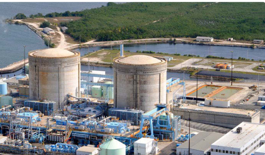
Turkey Point nuclear plant. (Image: FPL)
