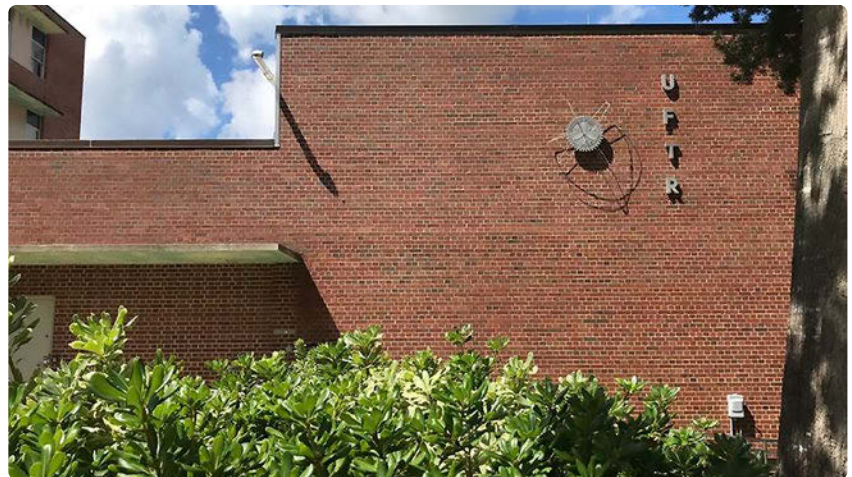
Signage on the University of Florida’s training reactor (a TRIGA reactor) building at its Gainesville, Fla., campus. (Photo: University of Florida)
