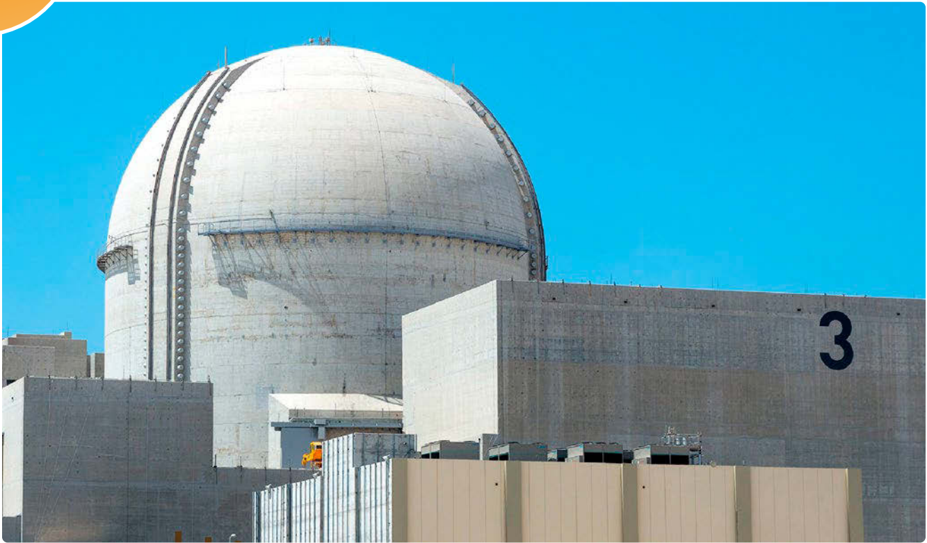
Barakah-3. (Photo: Nawah Energy Company)
