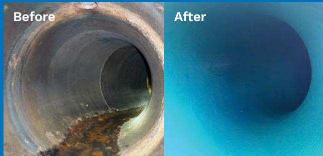
With structural capacity and a 50-plus year design life, Framatome's liner solutions will solve buried pipe aging challenges while taking you to the end of your plant's lifespan, helping what's buried - stay buried.
