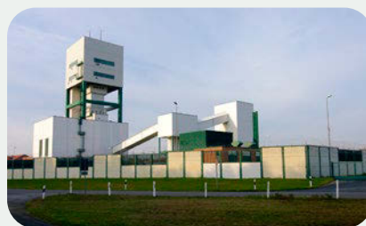
The headframe and buildings at the Gorleben salt dome in Germany. (Photo: Wikimedia Commons)
