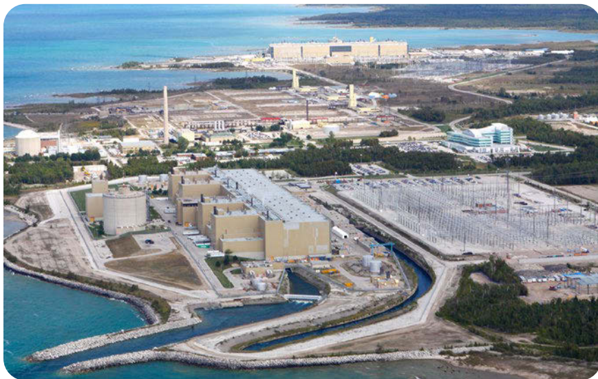
The Bruce nuclear power plant in Ontario, Canada. (Photo: Bruce Power)
