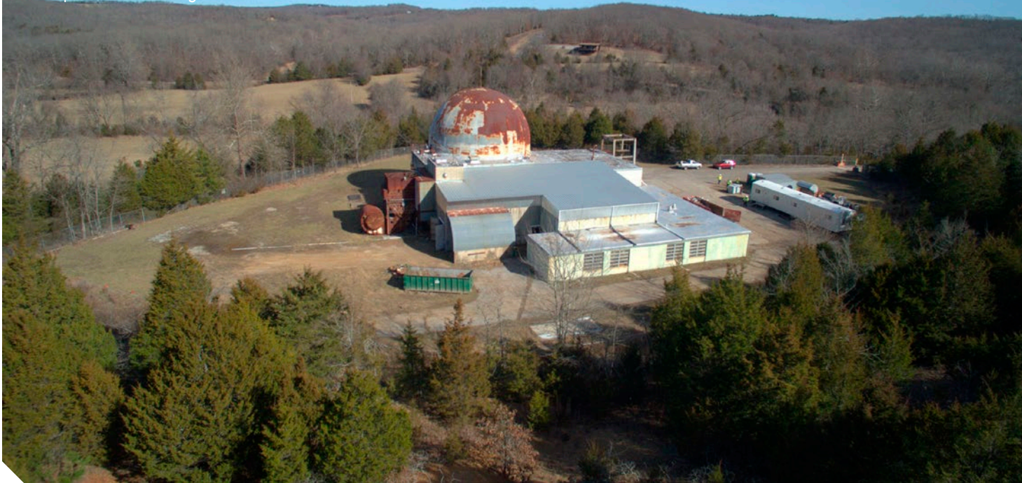
The SEFOR site in northwest Arkansas before decommissioning. The 20-MWt experimental fast breeder reactor used MOX fuel and liquid sodium cooling.
