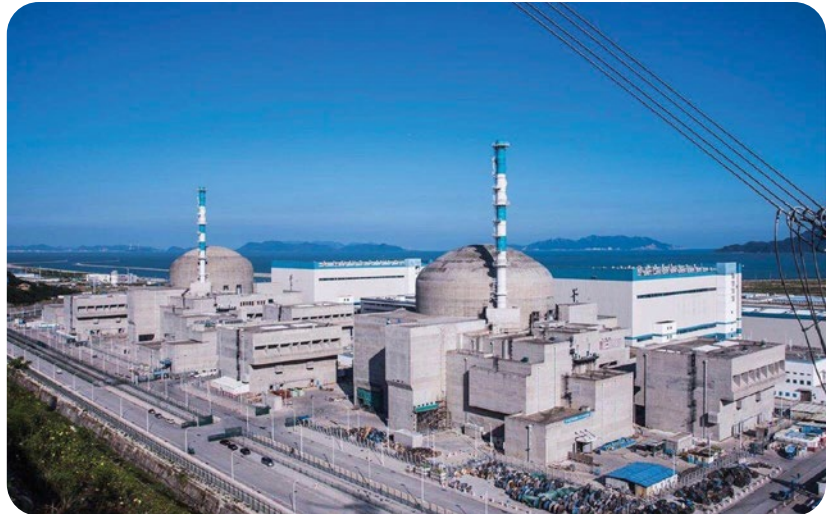
The Taishan nuclear power plant, in China’s Guangdong Province. (Photo: EDF Group)
