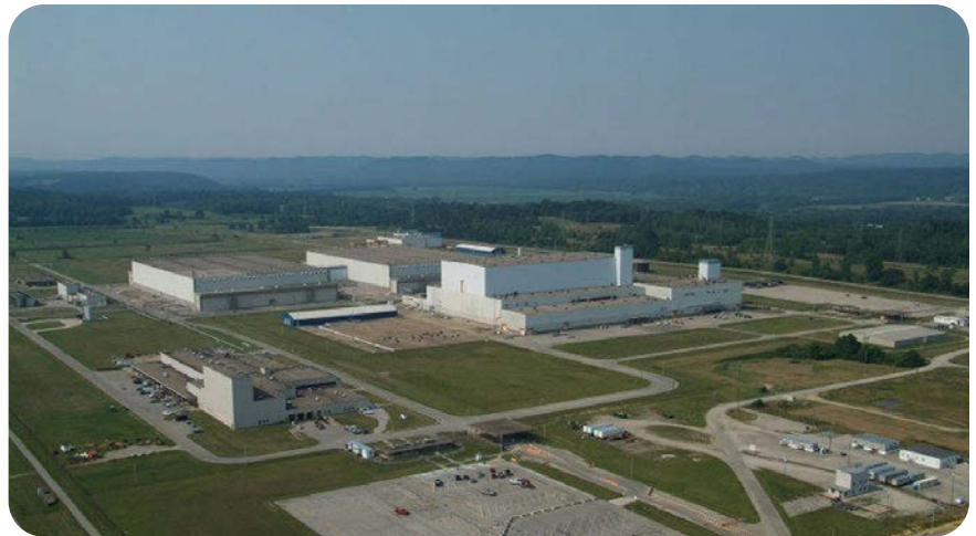
Centrus's American Centrifuge Plant, in Piketon, Ohio. (Photo: Centrus Energy)
