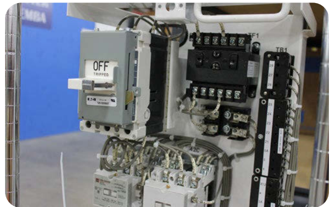
A motor control center sample bucket that goes into a motor control center. Having multiple components that make up this assembly and many subcomponents, it may be subject to parts quality testing.
