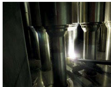
RADCAM Loki inspecting the top part of the thermal Sleeves
