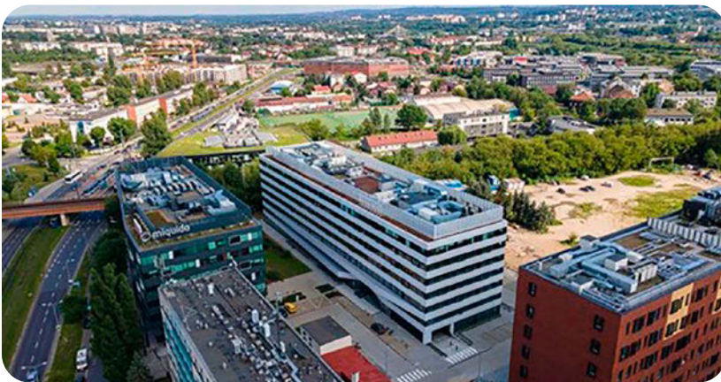
Kraków's Zablocie Business Park B. (Photo: OfficeMAP)
