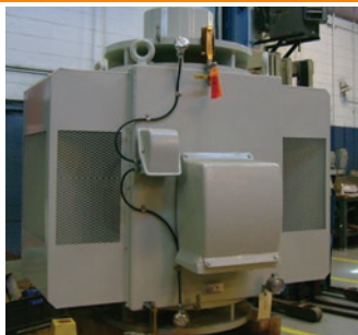
Safety-Related Motor Repair
