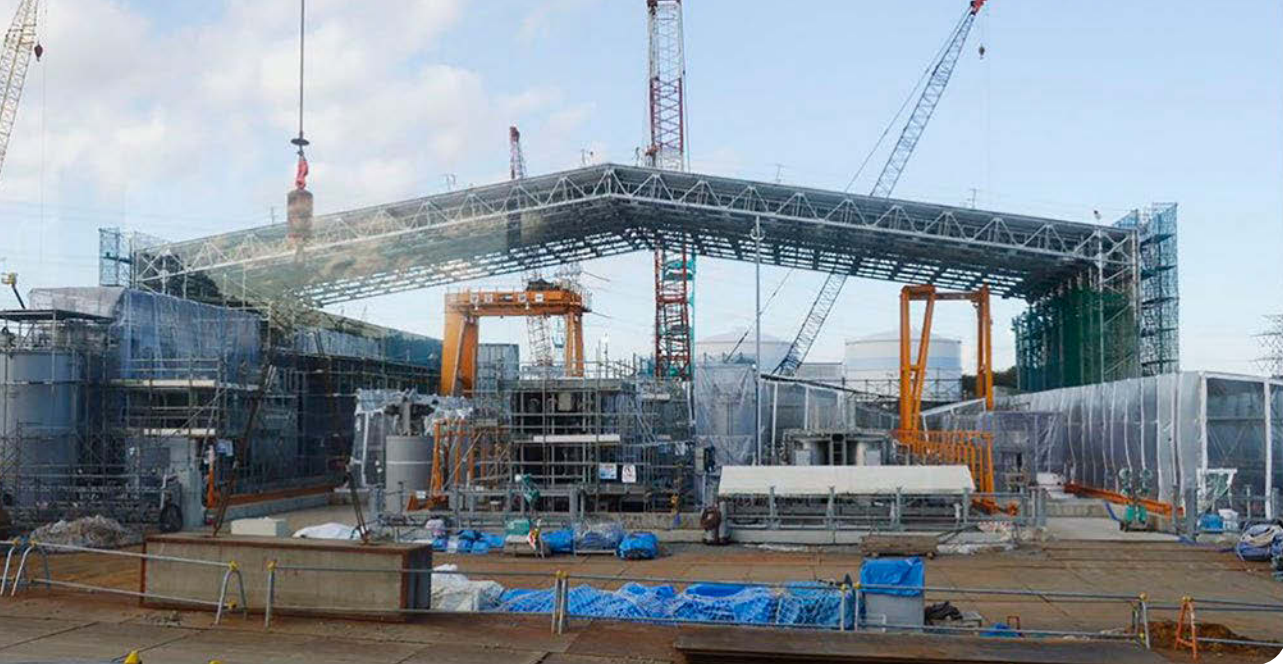
Construction of the ALPS processing facility on the Fukushima Daiichi site in 2013. Photo: TEPCO
