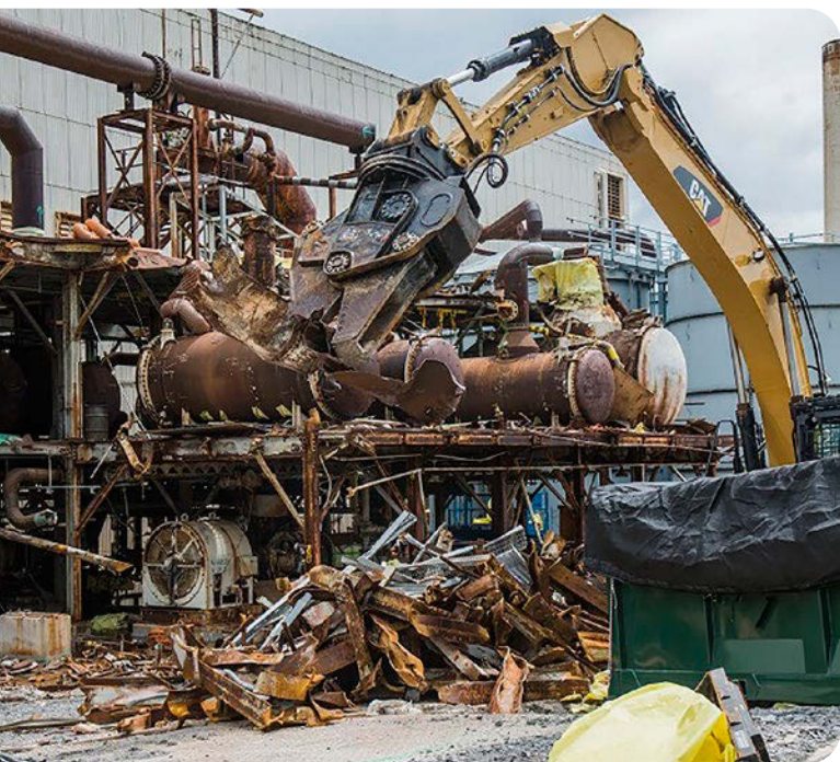
Crews cleaned and demolished COLEX equipment on the west end of the Alpha-4 building at the Y-12 National Security Complex. Photo: DOE
