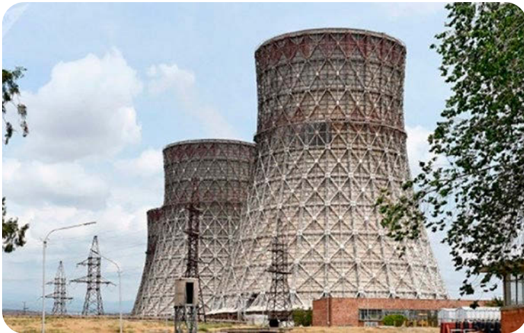
Cooling towers at the Metsamor nuclear plant. Photo: ANPP
