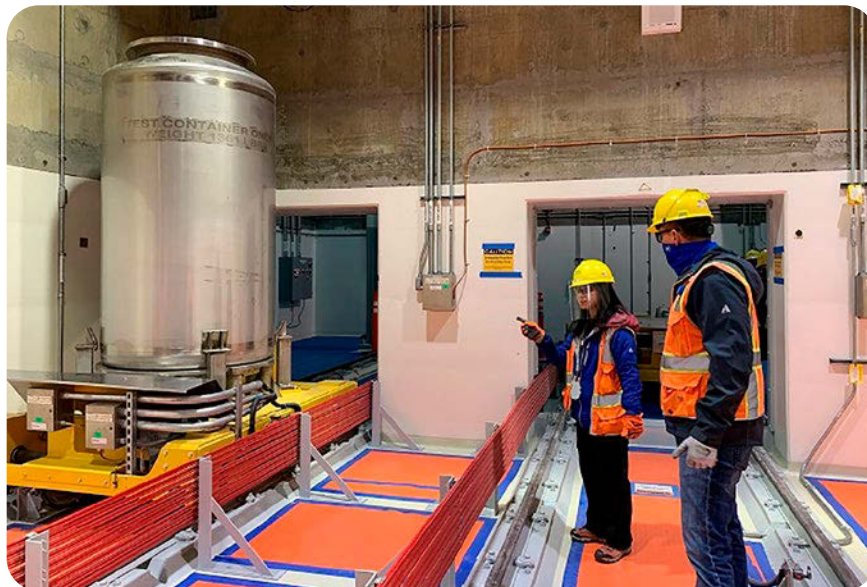
Hanford workers discuss LAW Facility mechanical equipment testing on the two units that make up the "bogie" transport rail system. Photo: DOE
