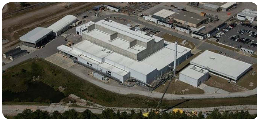
An aerial view of the Salt Waste Processing Facility at the Savannah River Site. Photo: DOE
