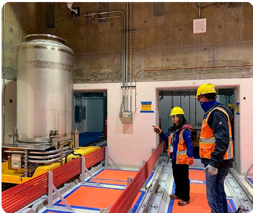
Hanford workers discuss LAW Facility mechanical equipment testing on the two units that make up the "bogie," or cart transport rail system. Photo: DOE
