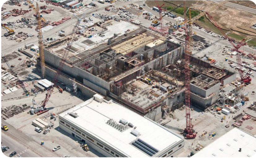
The MOX Fuel Fabrication Facility under construction in 2012. Photo: NNSA
