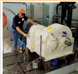
Gearbox Repair, Testing and Replacement
