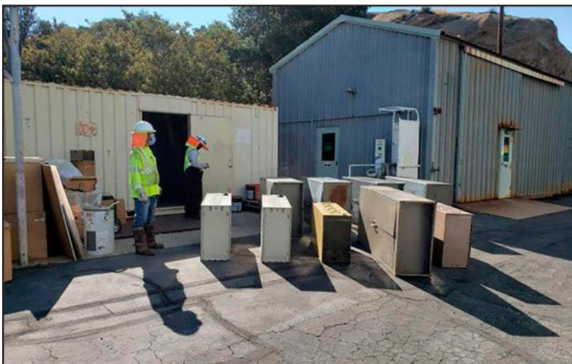
Workers from DOE contractor North Wind gather furnishings taken from buildings that are being demolished at the Energy Technology Engineering Center, part of the Santa Susana Field Laboratory in California. Photo: DOE
