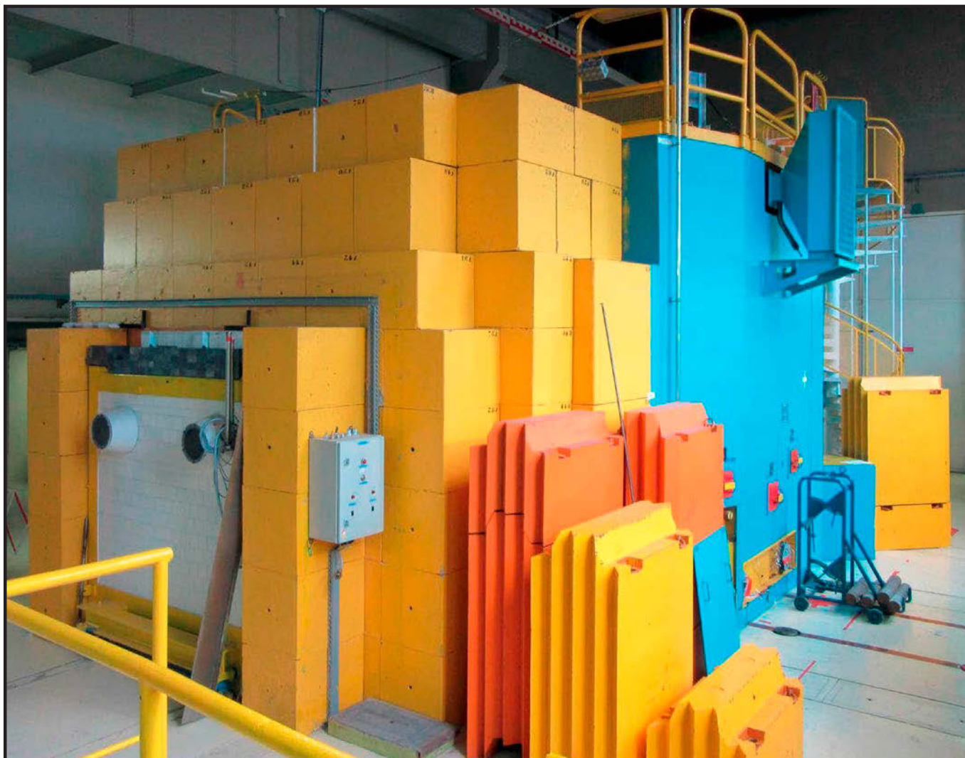
Ulysse reactor before dismantling. Photo: Orano
