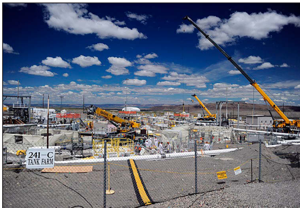
The C Tank Farm at the Hanford Site near Richland, Wash. Photo: DOE
