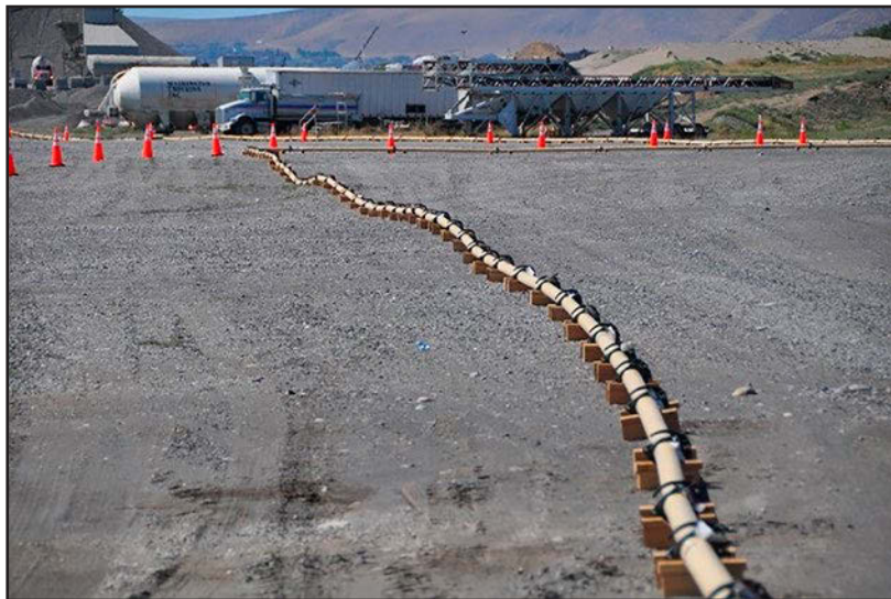
The DOE and CHPRC test a conveyance system that will pump engineered grout to three underground at-risk structures at the Hanford Site. Photo: DOE
