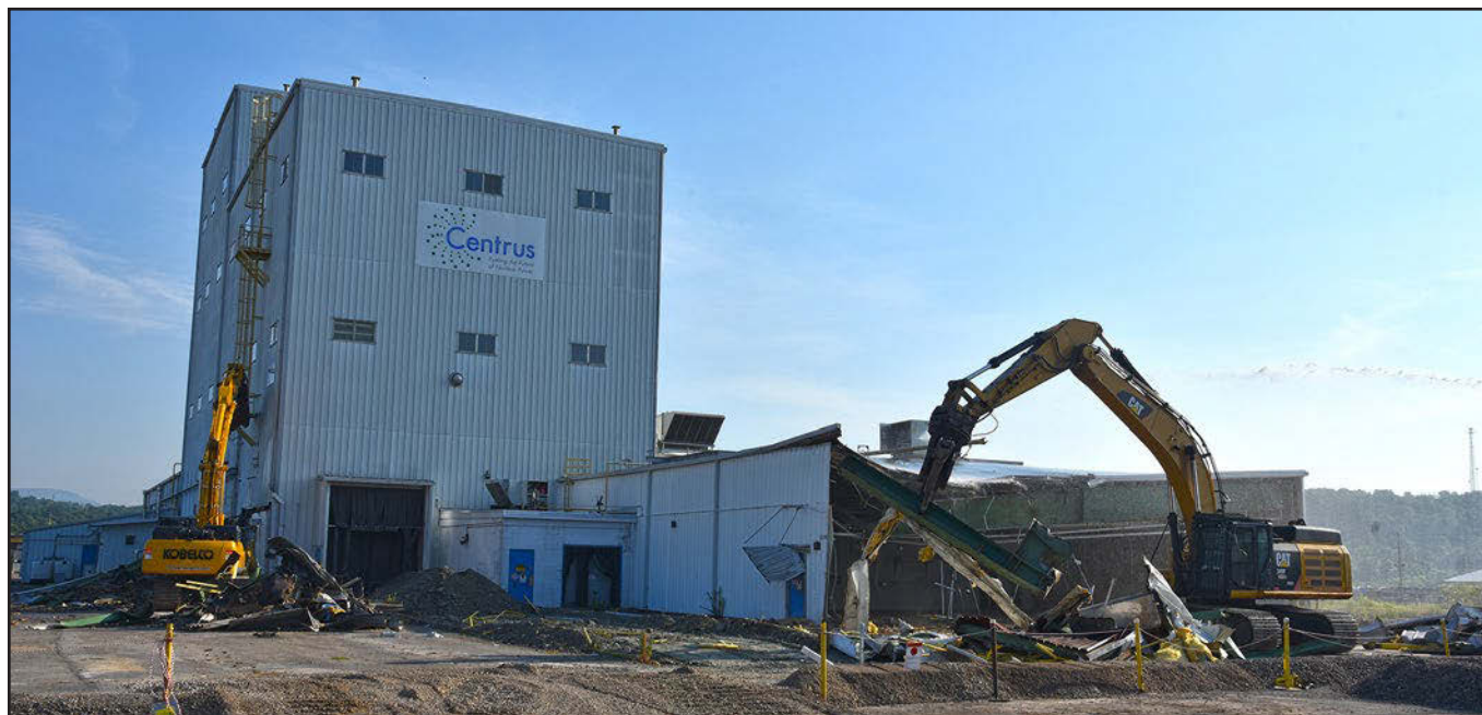
Demolition begins on Building K-1600 at Oak Ridge's East Tennessee Technology Park. Photo: OREM
