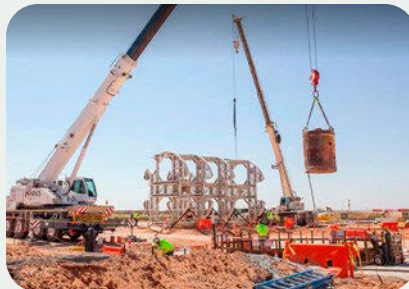
A bucket of dirt is lifted out of the utility shaft that is being excavated at WIPP. Photo: DOE OEM
